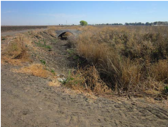
Photo 3. View looking downstream (east) toward the Mace Channel as it leaves the Project site. 7 October 2014.
