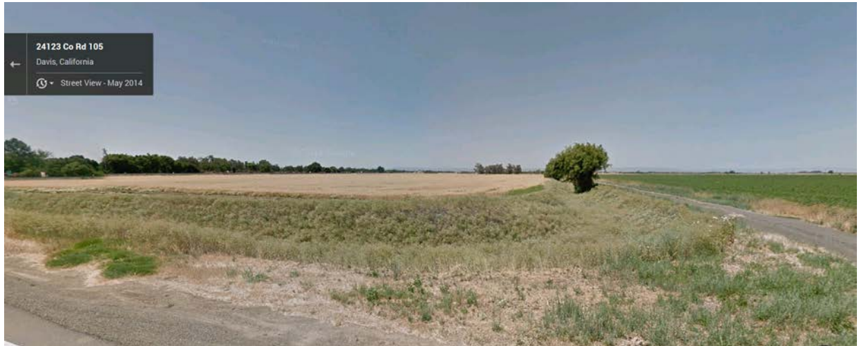
Photo 13. Google Street View, May 2014. View west from along Road 105 showing Mace Channel with no water present and ruderal weeds on bed and banks.
