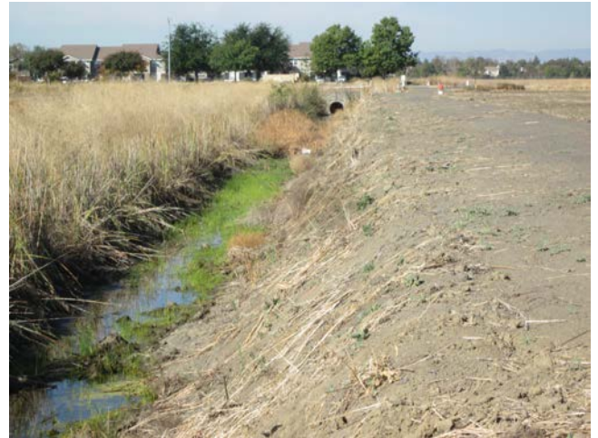
Photo 2. View west toward Mace Channel in western portion of site. Two adjacent culverts pass water beneath Mace Blvd., one of which is visible in distance. 7 October 2014.
