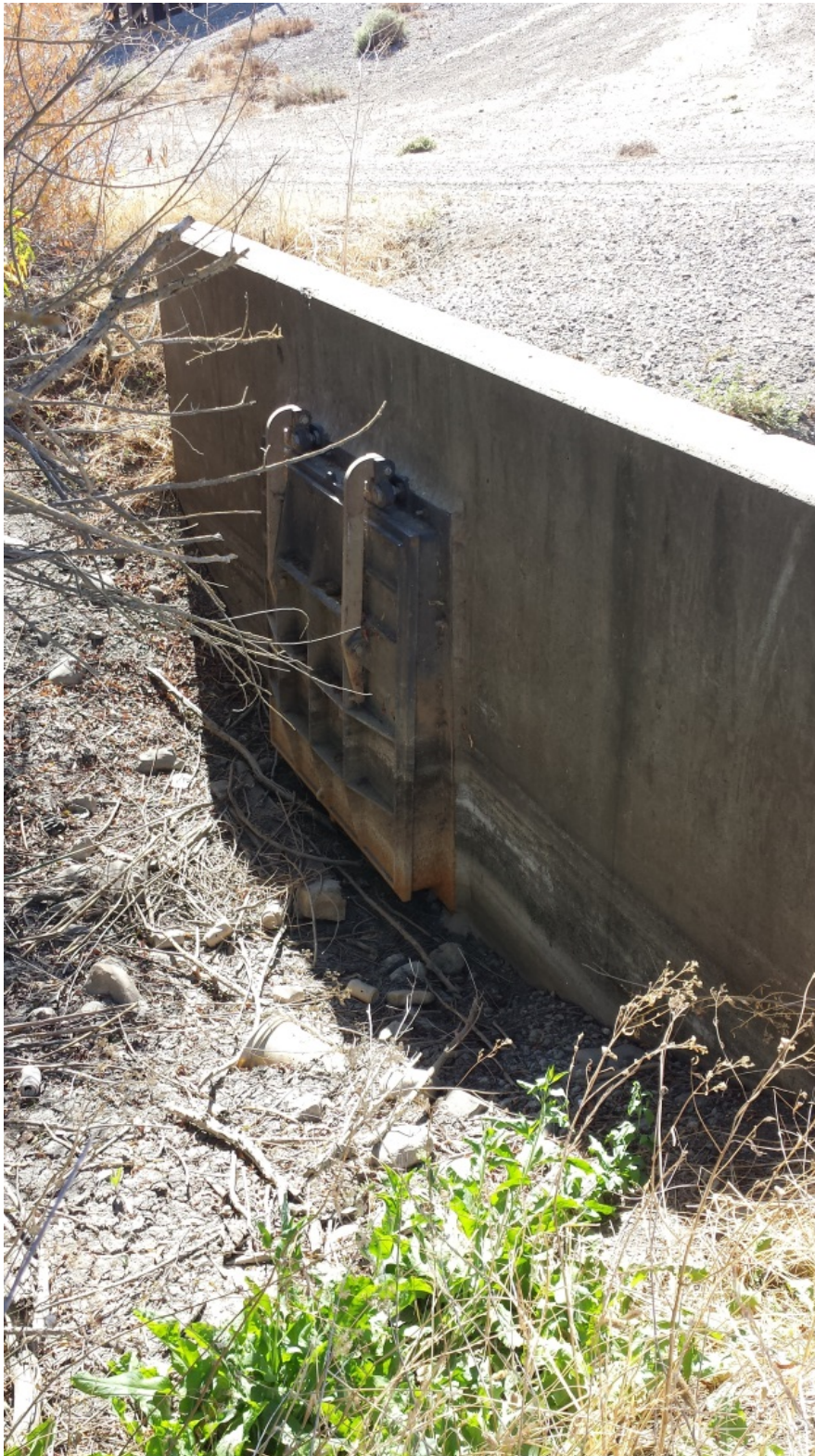
Photo 22. 7 October 2014. Mace Channel outlet, with large metal flapgate resting in closed position, on the Yolo Bypass side of the Yolo Bypass levee. No water is present.
