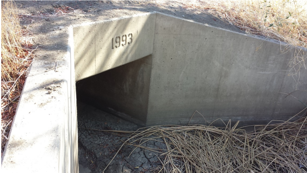
Photo 21. 7 October 2014. Mace Channel inlet under the Yolo Bypass levee. No water is present.
